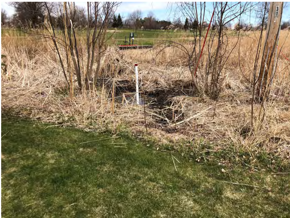
Photo 2 Downstream end of storm sewer draining N. Circle Drive. Ground surrounding storm sewer pipe is approximately 1.5' to 2' higher than pipe invert, causing a submerged condition.
