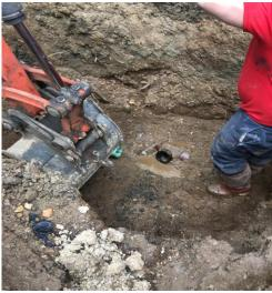
In the above picture, the white material at the bottom is grease removed from the resident's service line. The cost to have the line dug up and cleaned is the responsibility of the homeowner. If this material ends up in the sewer main, then all residents foot the bill to have it cleaned and removed.
